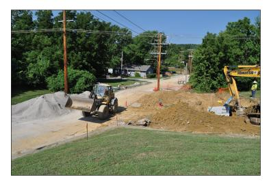
Thornton Street: This \$5 million project continued throughout the pandemic. It is still on schedule to be completed by the end of 2020. Work in the summer and fall included a reinforced concrete box culvert near the Municipal Service Center, tearing out existing street and roadbed from 10th Avenue to Maple Street and placing aggregate base for the street.
