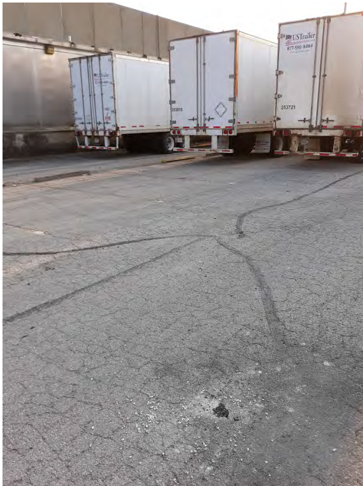
Photo 2: Abandoned Boring PB-1A; view to southwest.
