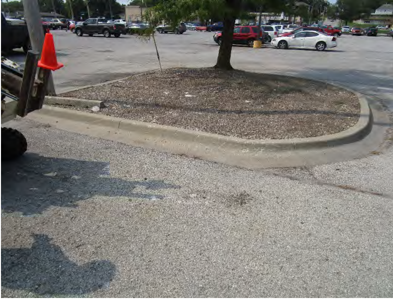
Photo 7: Installation of Boring PB-4 in southwest corner of the Subject Site; view to southwest.
