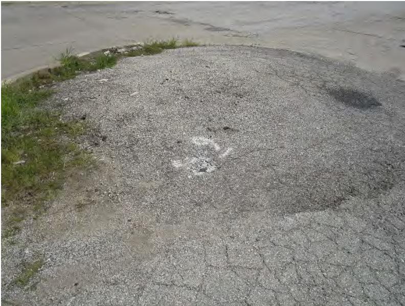
Photo 16: Installation of Boring PB-9 west of South 3 rd Street along southern boundary of the Subject Site; view to southeast.
