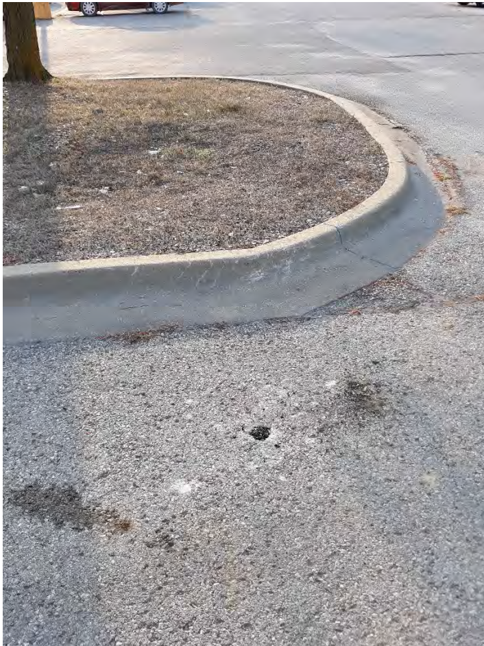
Photo 8: Abandoned Boring PB-4; view to west.
