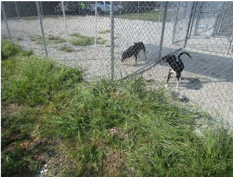
Photo 12: Installation of Boring PB-7 east of dog runs; view to southwest.
