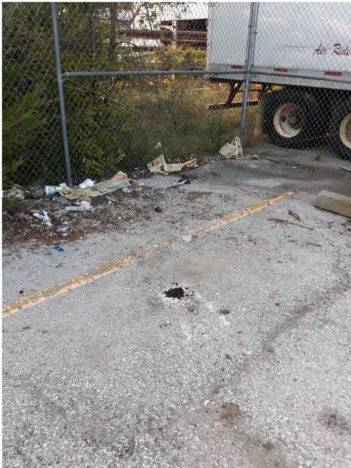
Photo 10: Abandoned Boring PB-5; view to northwest.
