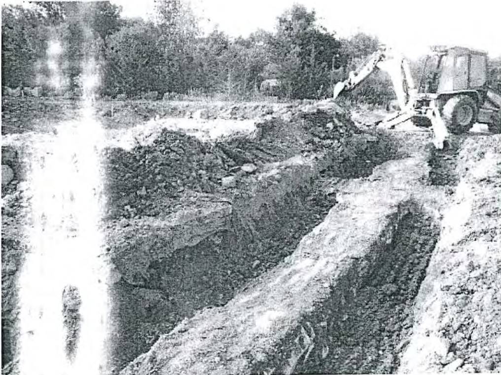
Existing excavation, looking southeast
