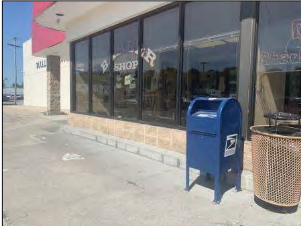
Northeast- View of the barber shop located onsite.
