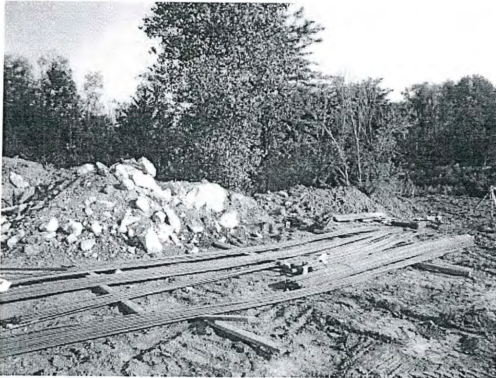
The rebar that was delivered this morning
