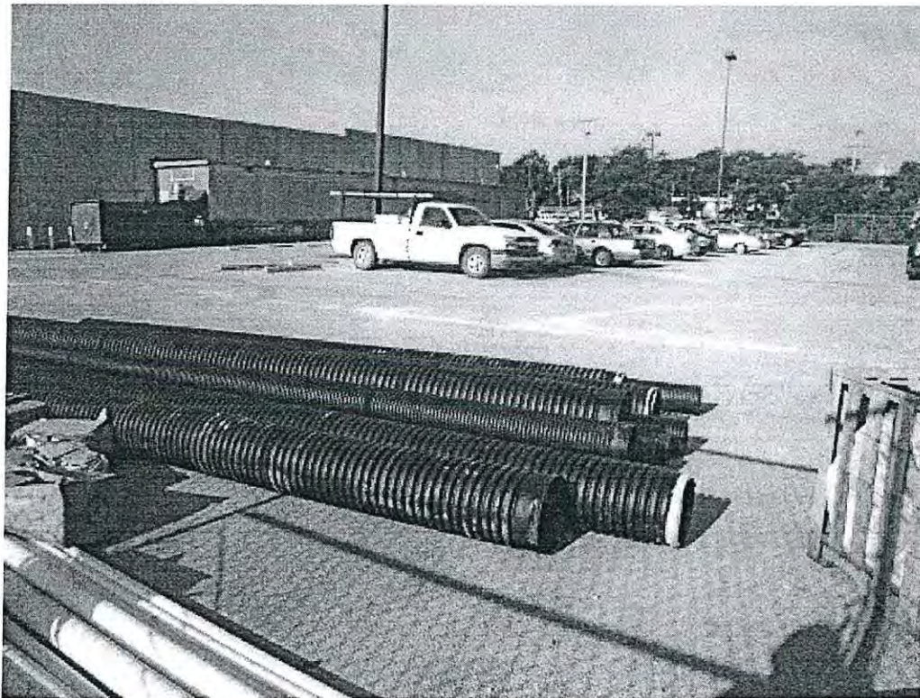
Additional stored plumbing supplies
