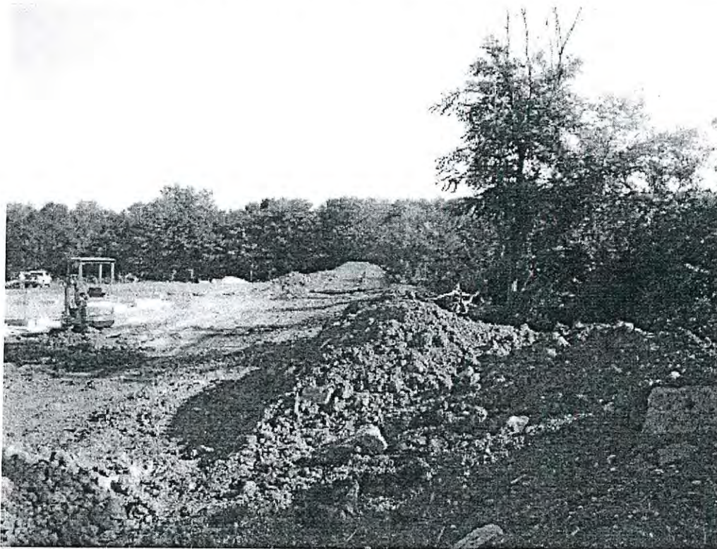
View looking north along the east construction limits
