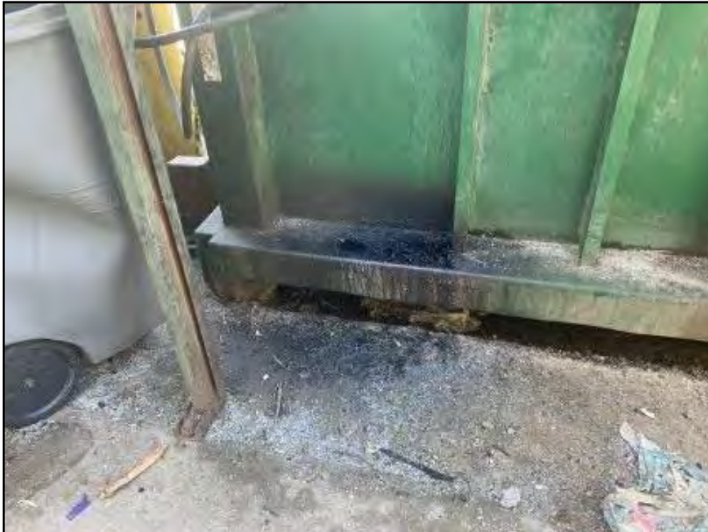
North- View of the de minimis spill observed in connection with the hydraulic trash compactor.
