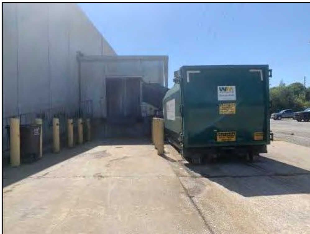
West- View of the hydraulic trash compactor on the north side of the structure.
