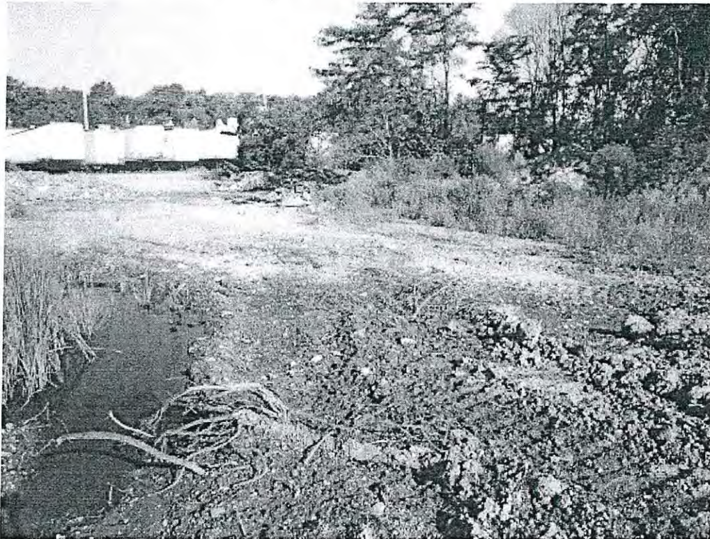
Standing water that had tank spillage in it, none was noticed during this site visit but noticeable after the tanks were relocated along the property's west edge (see past field reports for tanks temporary location on-site, also note dirt piles in the background which are from the Water Department's waterline trench
