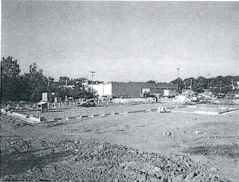
View looking southwest towards the building
