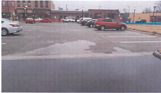
Pervious concrete pavement is a portland cement-based, rigid permeable pavement that serves not only as the surface layer of a stormwater management system, but also as a vital part of a water filtration system.
