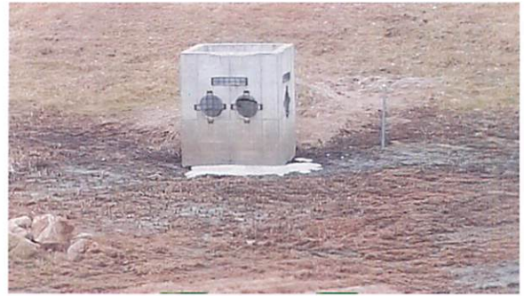
Basin Outlet Structure
