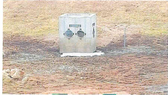
Basin Outlet Structure
