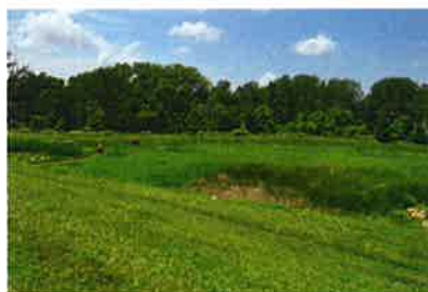
Contractors conduct annual maintenance of a detention basin near Leavenworth Walmart 5000 10 th Avenue in 2016 following a public meeting with City staff about best practices for managing detention basins.
