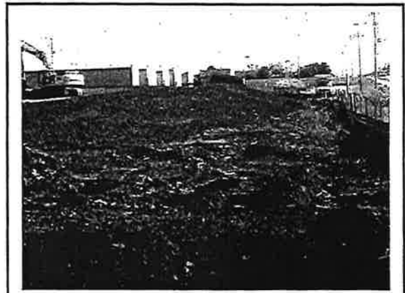
3. Looking east along south site boundary.
