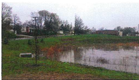
Eagles Hall Detention Basin After a High Rate of Rain
