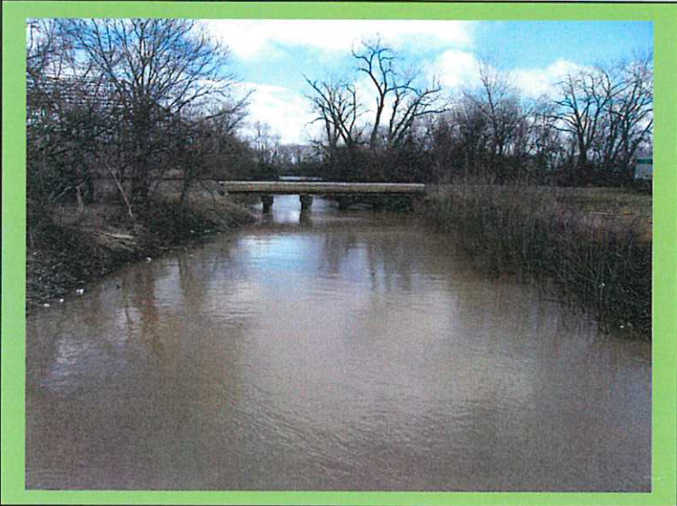
FIVE-MILE CREEK EAST LOOKING EAST (DOWNSTREAM)
