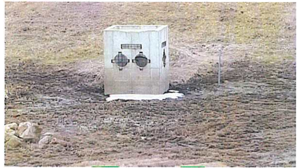
Basin Outlet Structure
