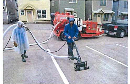
A Hydro Excavator Modified to Vacuum Sediment From Pervious Pavement
