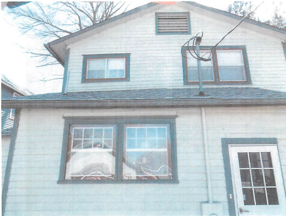
Replacement Windows 101, 102, 202 & 203 House North Side
