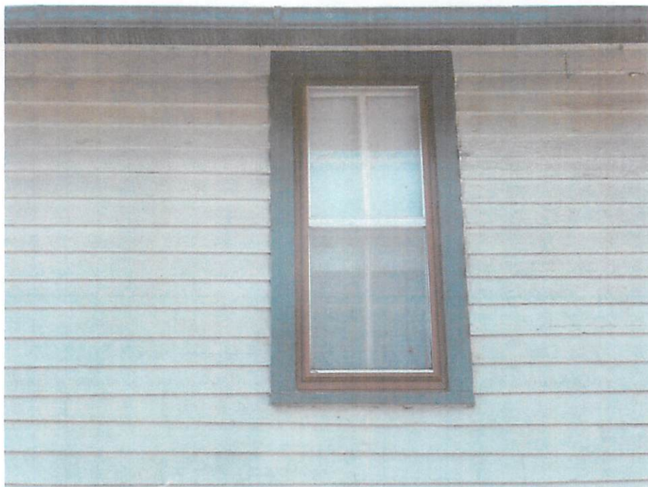
Replacement Window 204 East Side, 2 nd Floor
