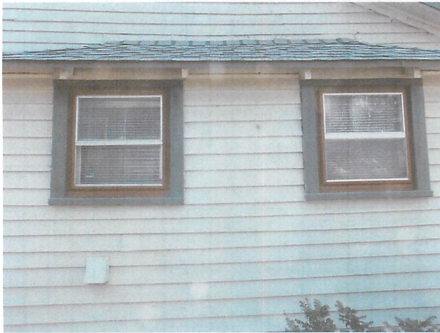
Replacement Windows 103 & 104 East Side, 1 st Floor
