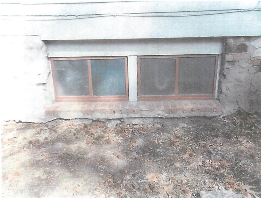
Replacement Window 501 Basement, West Side
