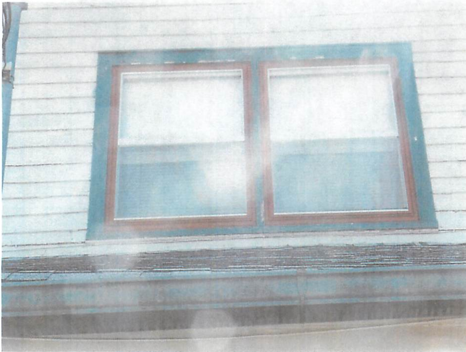
Replacement Window 202 North Side, 2 nd Floor
