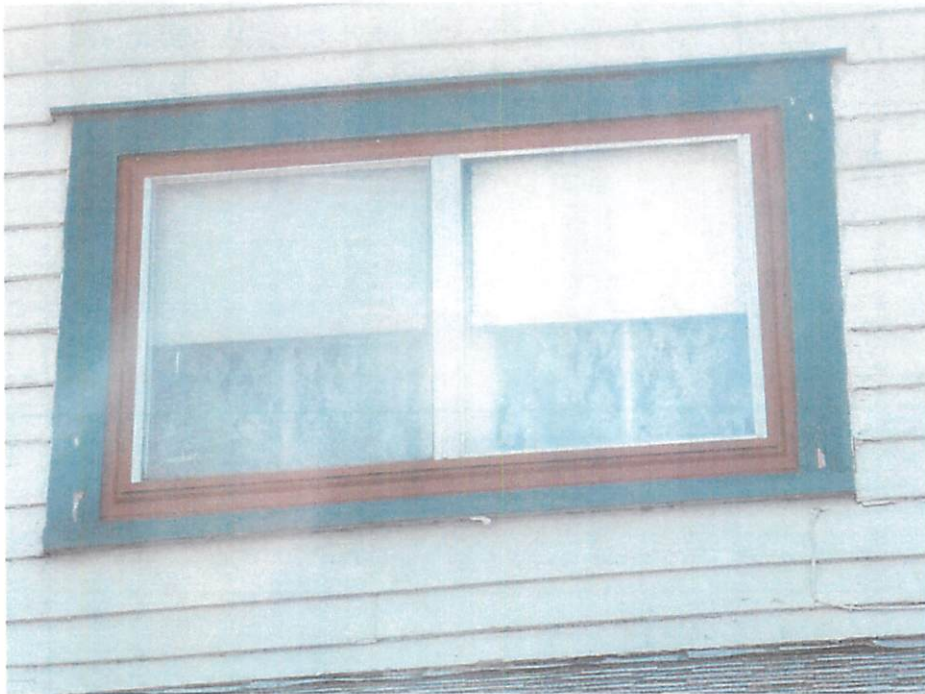
Replacement Window 203 North Side, 2 nd Floor
