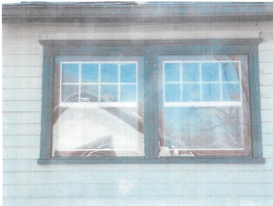
Replacement Windows 101 and 102 North Side, 1 st Floor
