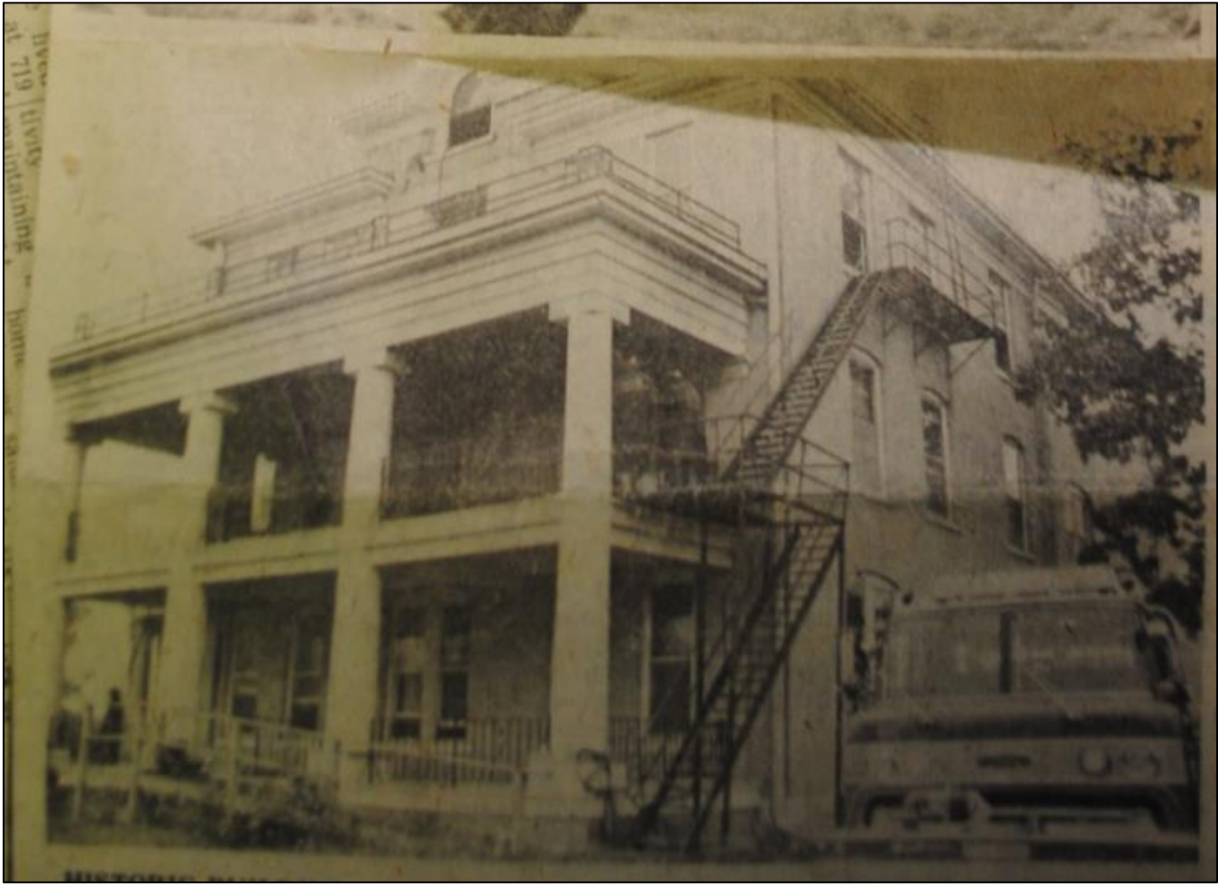
Figure 4. November 1983 image of the east elevation, showing the removal of decorative elements and the covering of the columns. Source: Debra Bates and L. Candy Robinson, "Fire Damages Small Building," The Leavenworth Times (8 November 1983): 1.
