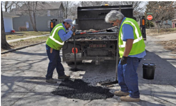
Public works employees repairing streets.
