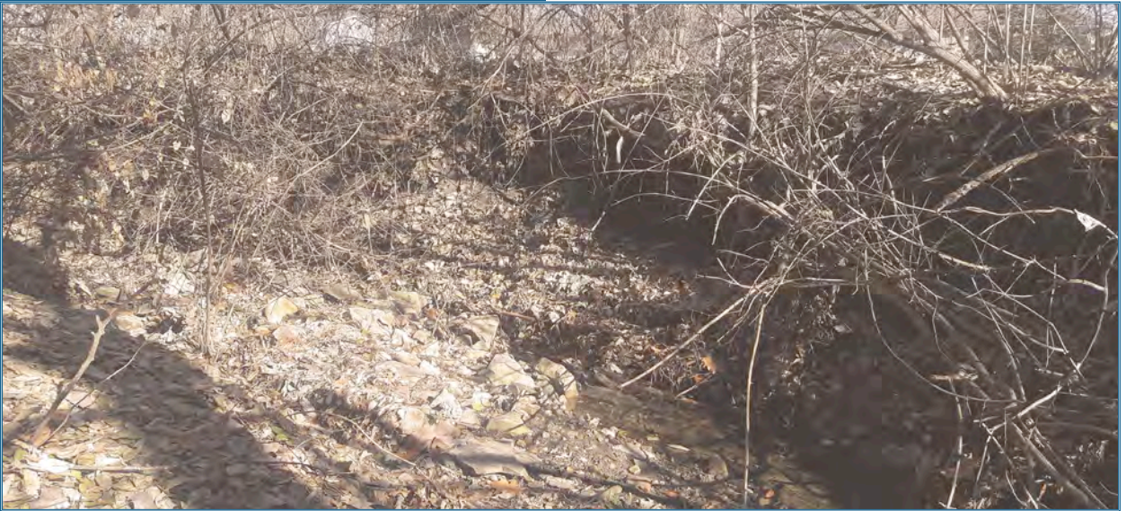
Figure 12. Vertical cut bank in Reach 2
