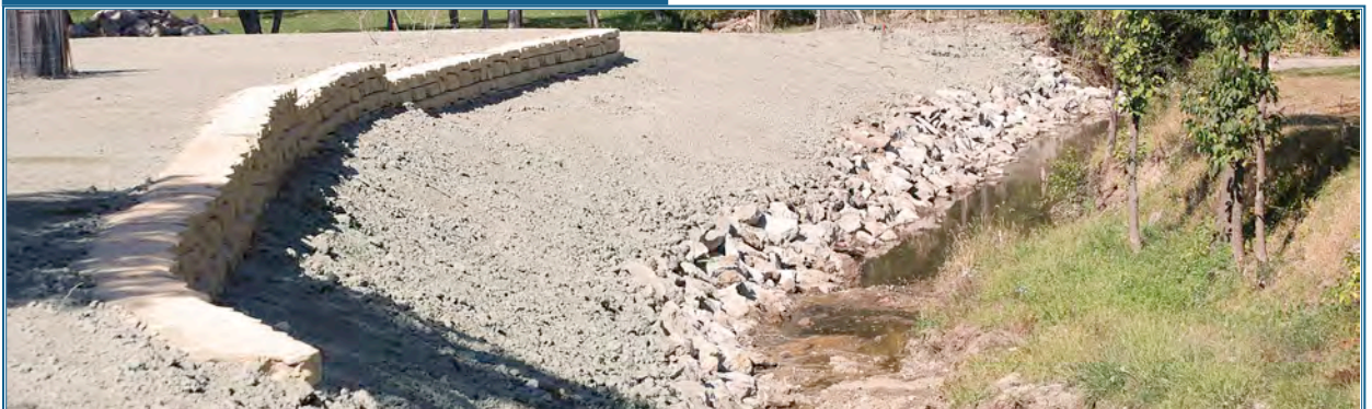
Figure 24. Peaked stone toe protection example
