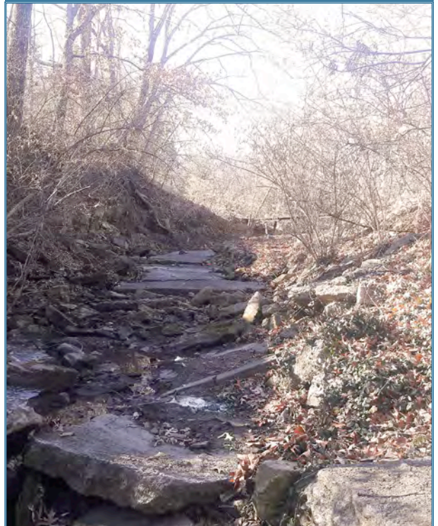
Figure 18. Concrete revetment, Reach 4
