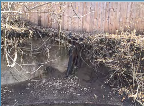
Figure 21. Bank slide failure behind residences, Reach 6
