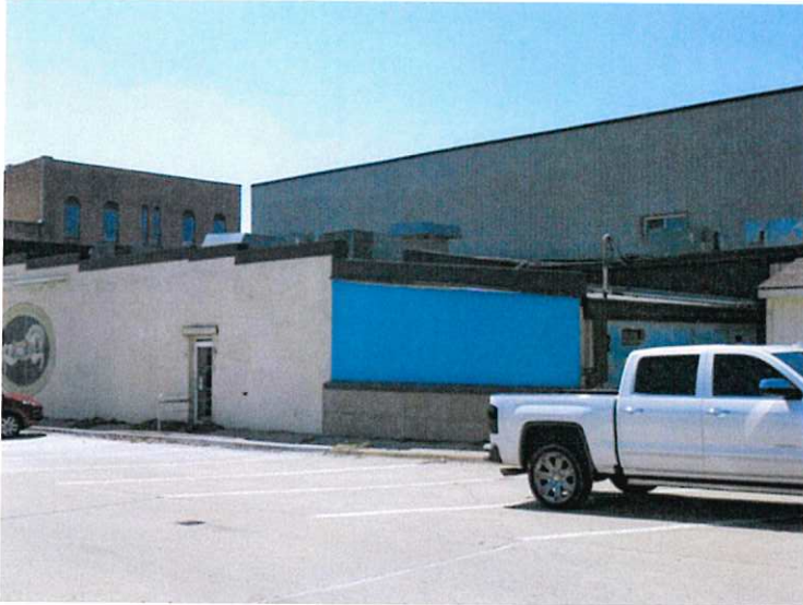
3. Building as seen from the northeast.
