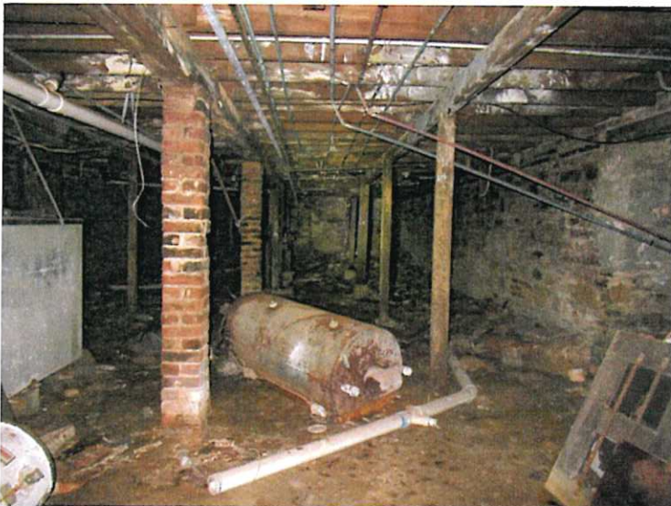
10. Looking south in the eastern half of the basement.
