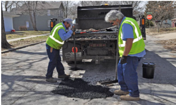
Public works employees repairing streets.
