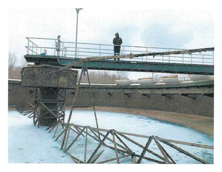
Comment from inspection: "While the mechanism is beyond it useful life, the bridge however is in remarkable shape and could be reused."
