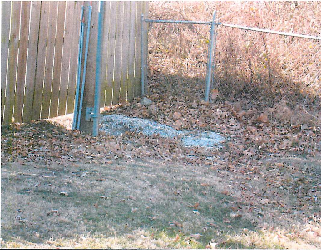
#3: The Southwest corner of 1106 South 14th St. Water from the woods and neighboring yards directly south enters this portion of the yard
