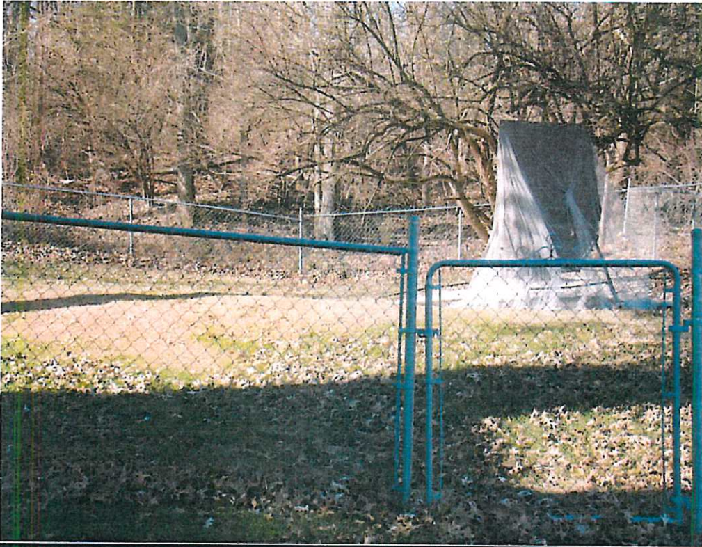
#1: Northern side of 1106 S. 14th St Hidden Point Subdivision. Current owner Melvin and Judy Watson Note the slope of the fenceline on the western edge of thier property
