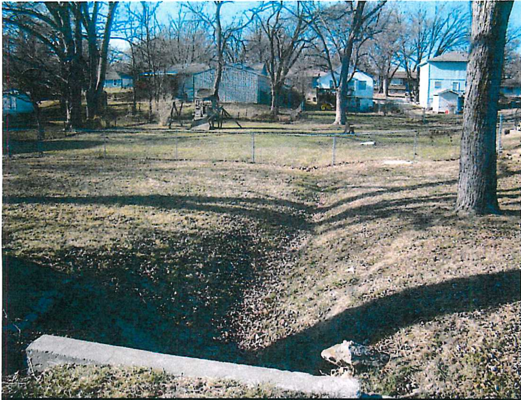
#11: Water from Madison St continues to flow eastward into this area adjacent to 910 Washington St. During periods of continuous rainfall this area floods
