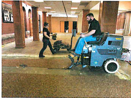
New Floor in Riverview Room
