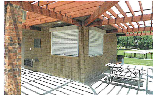
Cody Restroom Overhang
