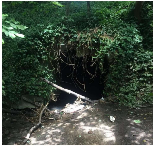
Figure 3: 72" Stone Arch Inlet in Open Channel, Looking Northeast
