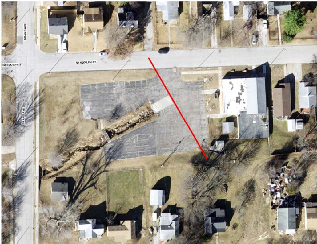
Figure 4-3 Randolph Street Culvert Overtopping Results Location
