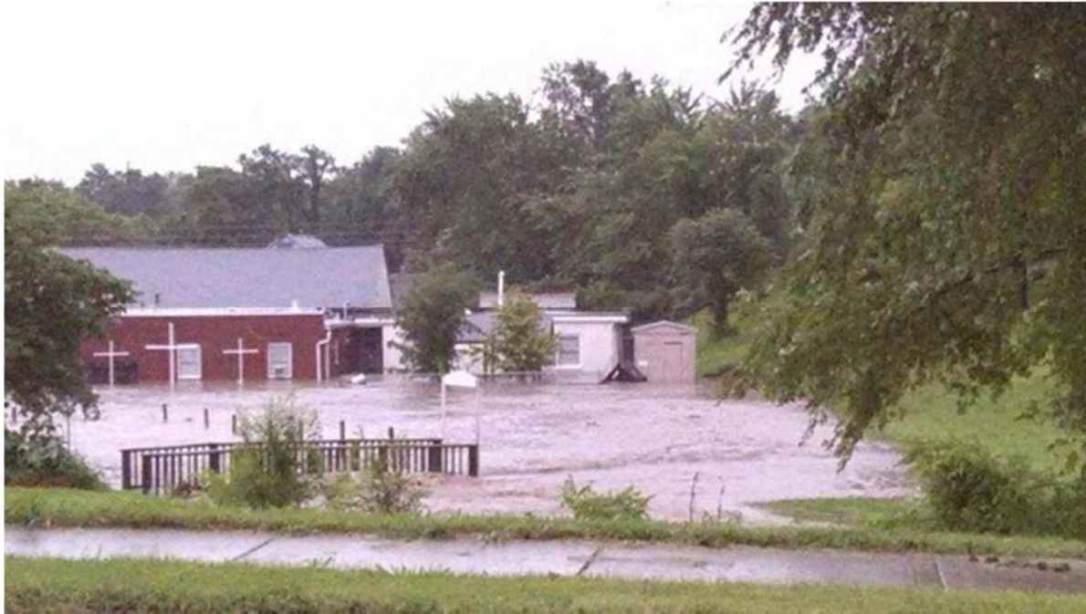
Figure 1-1 Historic Flooding of Rock of Ages Church on July 6th, 2015 (source: City of Leavenworth, Kansas)
